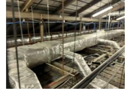
Attic - Ventilation Ductwork
